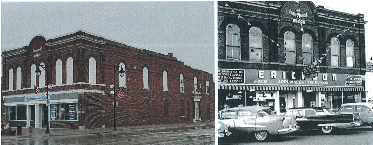
Left: Existing façade showing mothballed upper floor windows and infilled openings on the side elevation. Right: 1961 photo showing original windows and storefront design as "Erickson Appliances, Television"
