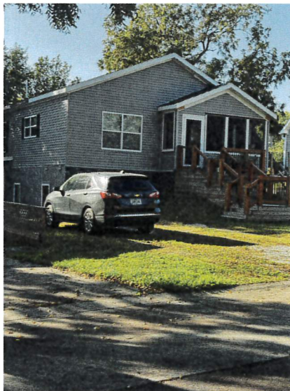
Property rebuilt (rebuild at owners' expense; not covered by the program)
