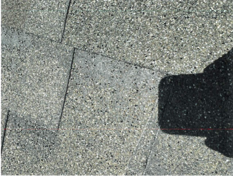
South Side (Fiberglass showing on entire shingle) (Estimated 0-1 Year of life left in shingles on South Side)
