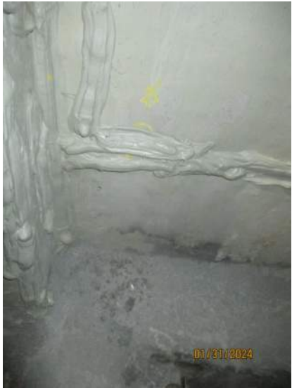
After Repair (fillet was already placed before the after repair photo could be taken)
